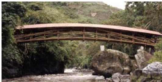
bamboo bridge, popayan colombia, fig.3 Jörg Stamm, 1997
