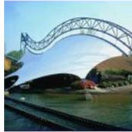
Cenotec steel trusses
