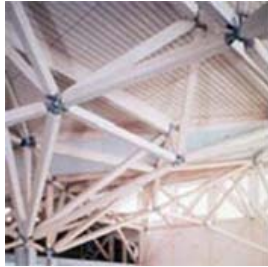
Arch. Brader wood structure
