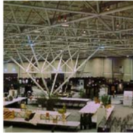
Technikon steel framework
